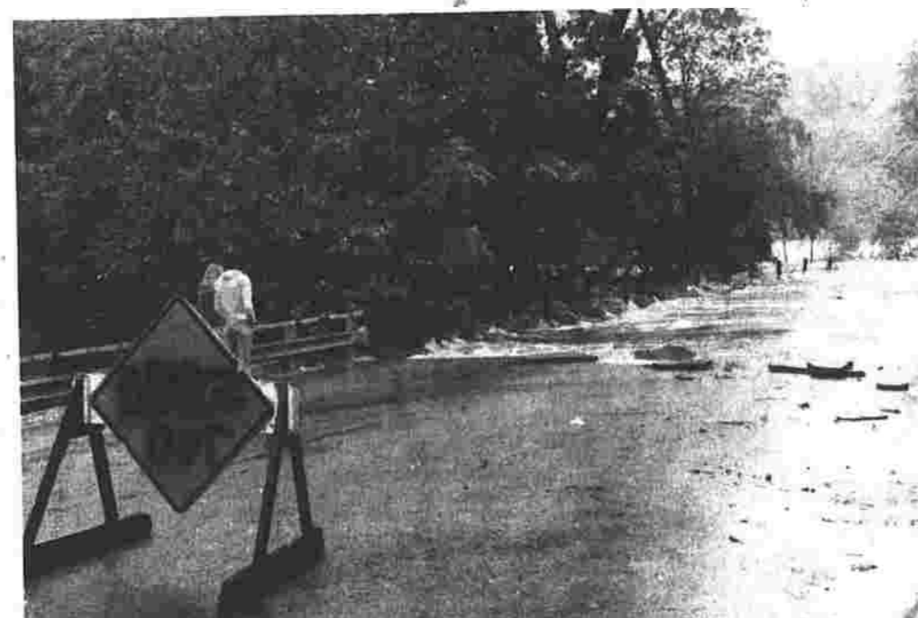
THE SIGN SAYS IT IN ANDOVER Bunker Hill Road suffered the most damage
